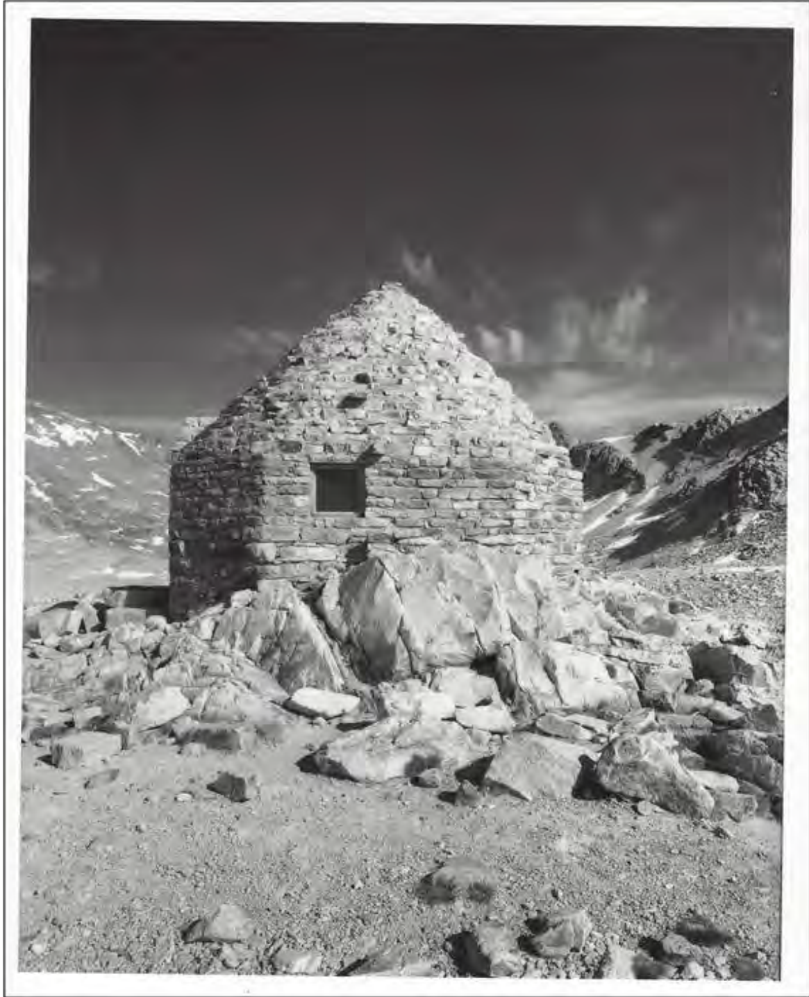
Photo 3. North side elevation showing window, 2015.
