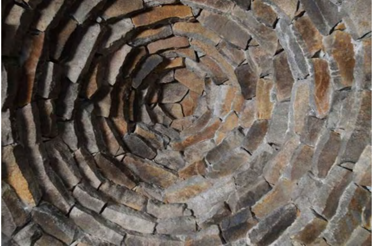
Photo 6. Corbelled granite conical ceiling detail, 2015.
