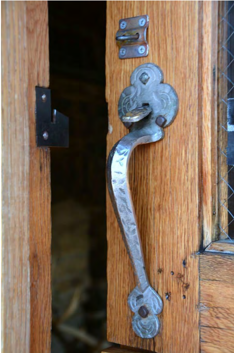
Photo 10. Arts and Craft Style hammered entry door pull and latch, 2015.
