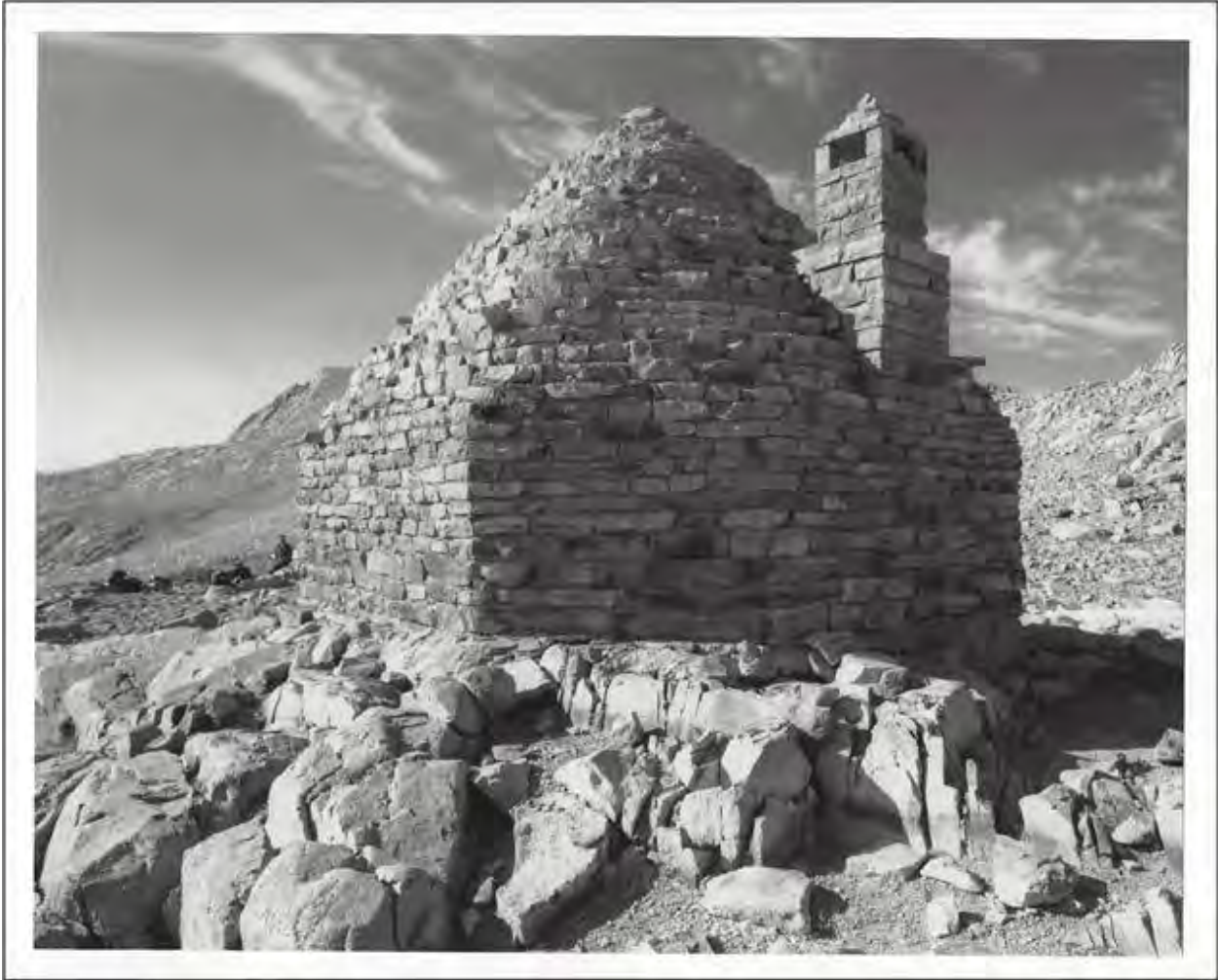
Photo 2. South side elevation showing chimney, 2015.
