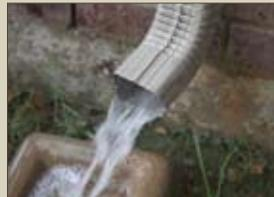
*Downspouts that flow into yards can reduce stormwater overloads*
