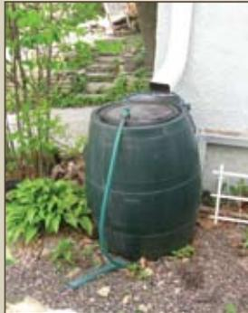
*Rain barrels can store rainwater and keep it out of drains.*
