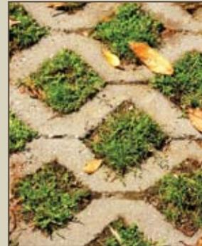
*Permeable pavements allow rain to seep into the ground*
